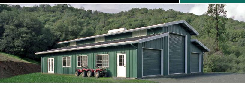
PBR Panel is an economical, structural, through-fastened roof and wall panel suitable for general usage.
